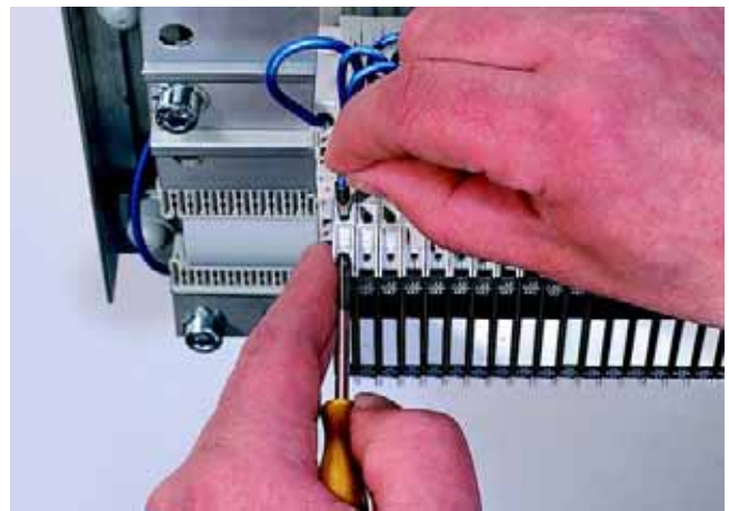
Connecting a lead to the spring-loaded terminals
